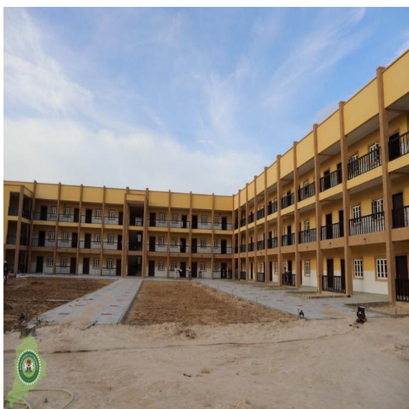
Figure 2: One of the ten Mega Schools Constructed by the Borno State Government in Jere LGA
